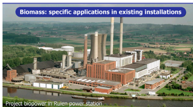
Figure 22. Electrabel Ruien power station
