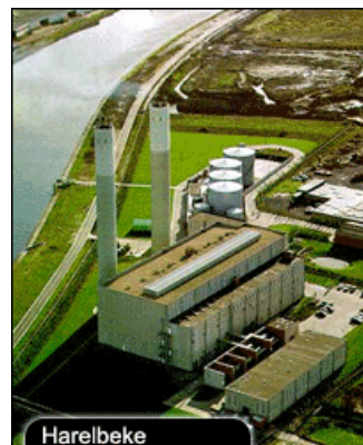
Figure 17. Harelbeke power plant os SPE.
