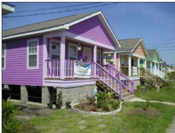
Houses with pier foundations recently constructed by Habitat for Humanity in New Orleans, LA.
