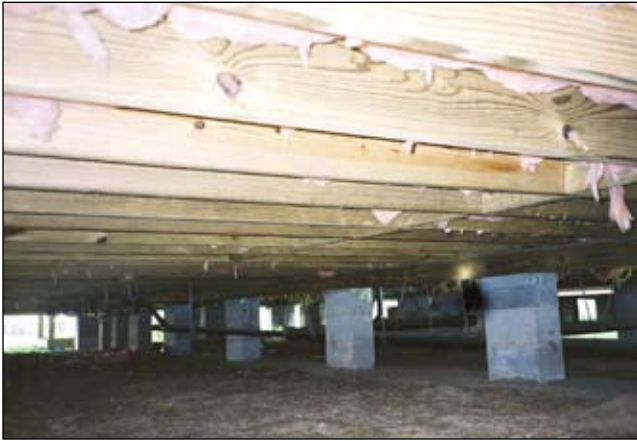
This pier foundation supports a raised floor framed with pressure-treated lumber.
