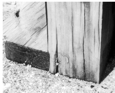
Figure 23. This poor method of assembly will allow water to wick into the end-grain of this treated post near the ground. Stain has already developed near the ground contact region as a result of excessive water absorption. (Source: Forest Products Society)
