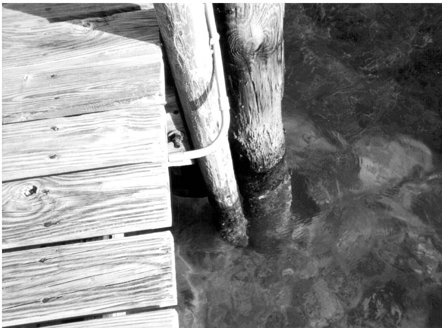
Figure 19. Utility poles and pilings in salt water require protection from marine wood borers. In some marine areas, the wood must be treated with an inorganic arsenical in addition to creosote.
