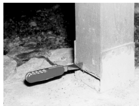
Figure 24. Inspection of posts is simply accomplished with a probe. (Source: Forest Products Society)
