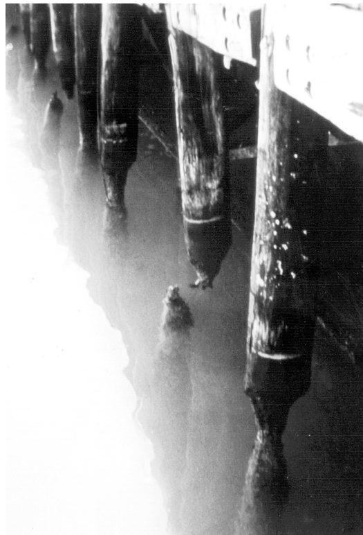
Figure 21. These boat dock pilings have been heavily damaged by marine borers, commonly known as gribbles (Limnoria). (Source: Forest Products Society)
