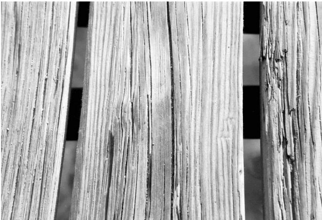
Figure 1. Severe weathering occurred on the surface of these treated southern yellow pine boards used to construct a boat dock. Most docks are continually exposed to wet and dry conditions and direct sunlight. It is recommended to brush apply each year a water repellent that also protects from ultraviolet (UV) degradation of the wood surface.
