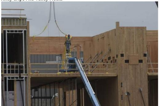
A worker with Andersen Construction rigs a CLT panel for lifting.
