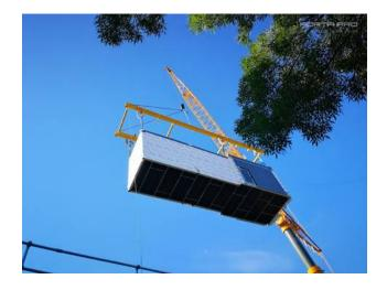
Onsite construction was completed in only two weeks without disrupting neighboring working clinical departments or blocking traffic pathways for ambulances. By assembling the modules in a factory, onsite dust and noise was mitigated as compared to traditional construction.
