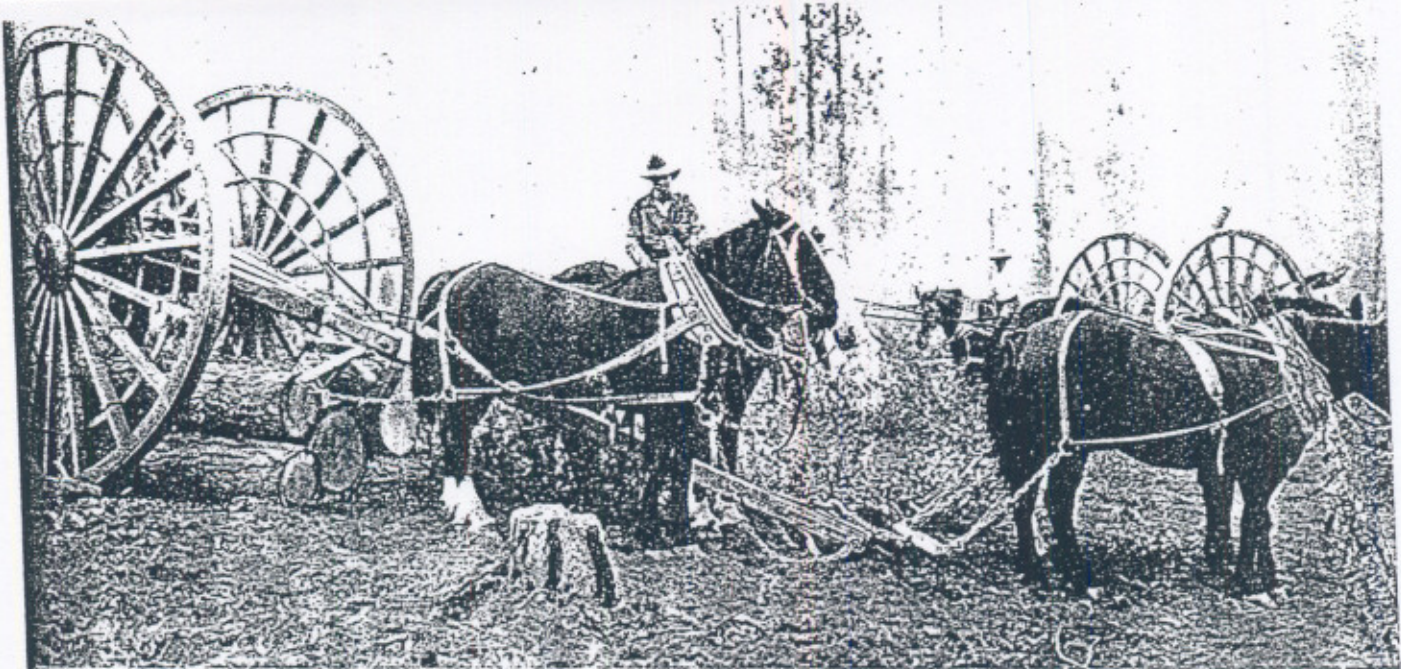
12 FOOT WHEELS AT BEND. Logs have been chained to hoisting rigging and lead team is ready to pull. These wheels were the slip-tongue type developed by Redding Iron Works. (Photo Paul Hosmer)
