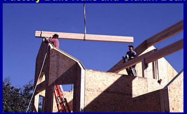
LVL(Laminated Veneer Lumber) and OSB factory built wall panels
